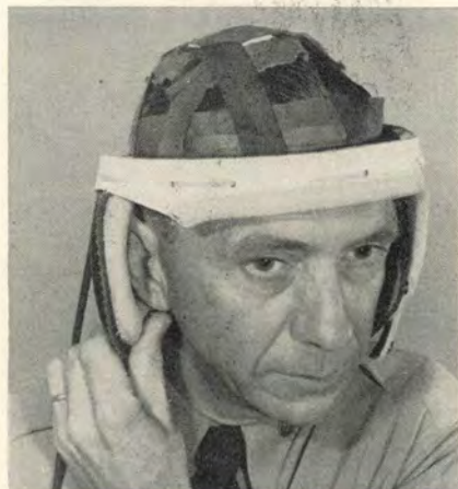
Earphone mounting pads should be adjusted to touch the lobes of the ears.
